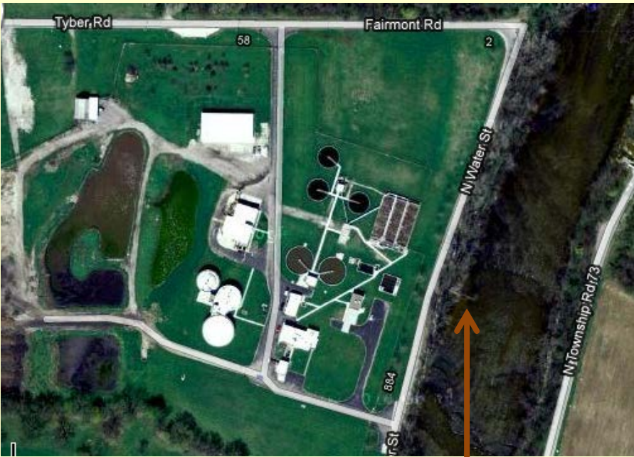
Tiffin sewage treatment plant with discharge pipe to the Sandusky River
